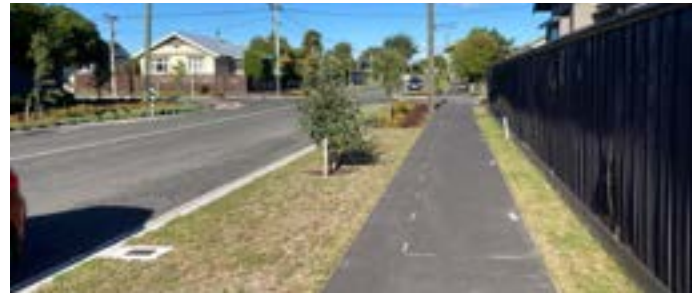
Randall St Post Rebuild
